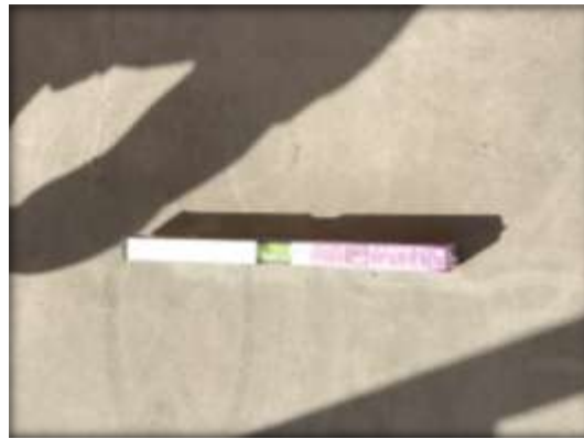
Fig 13: Adjusting Horizontally Steel Frame.
