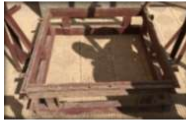
Fig 8: Supporting Steel Frame
