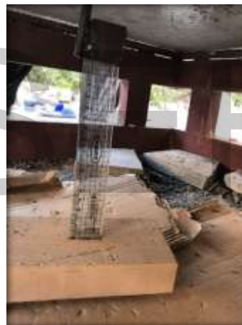
Fig 14: Placing Graded Ruler Under Steel Indicator.
